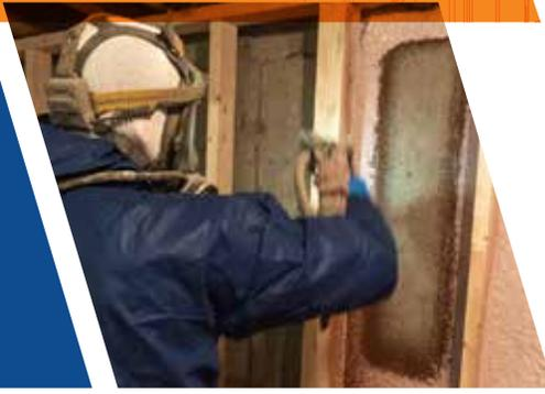
Spray Foam is a spray applied polyurethane insulation. 2lb medium density closed cell spray foam is our product of choice. It can be used on numerous areas of a building to prevent air leaks, condensation and mold growth, all while making the space more comfortable.
