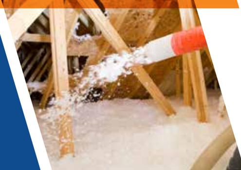
Fibreglass loose fill can be installed in your attic and is often the easiest and most cost-effective way to improve the efficiency and comfort of your building. Although it doesn't prevent air movement, it will increase overall insulation value.
