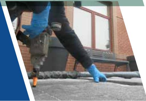
The process of raising and leveling concrete slabs has been around for years, but lifting and leveling concrete slabs using polyurethane foam is a game changer. The process is cleaner, faster and more environmentally friendly than any of the alternatives, and far more economical than replacing the concrete. With foam being lightweight, it will not compound existing problems of poor compaction.
