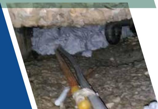
FillFoam is a product specifically designed for filling void spaces. This hi-density foam can be pumped in large quantities and over long distances to fill any void space and support the surrounding structure to prevent it from collapsing. FillFoam acts like a large sponge, absorbing moisture then releasing the moisture when the surrounding area dries out.
